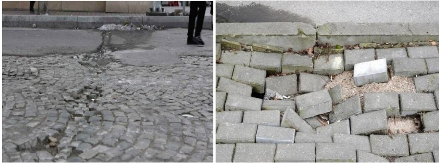
Fig. 1. Deformed pavements.
